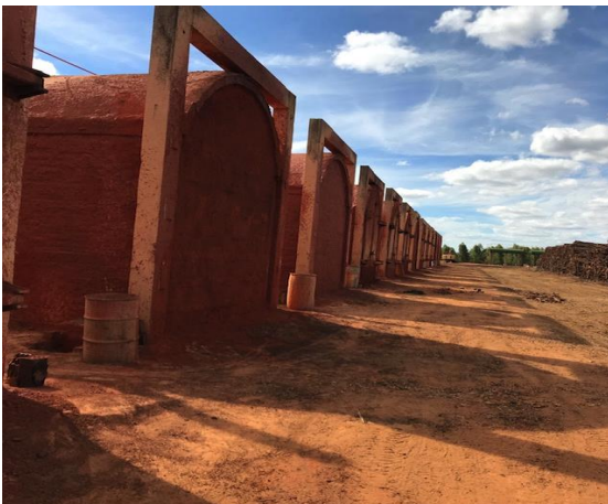
Large scale rectangular masonry brick kiln
