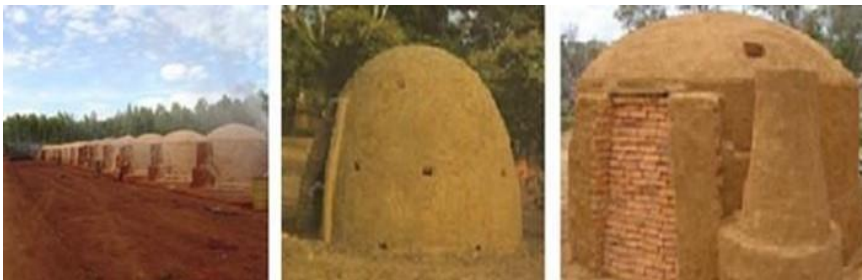
Figure 9 - Circular masonry brick kilns with partial mechanization.
