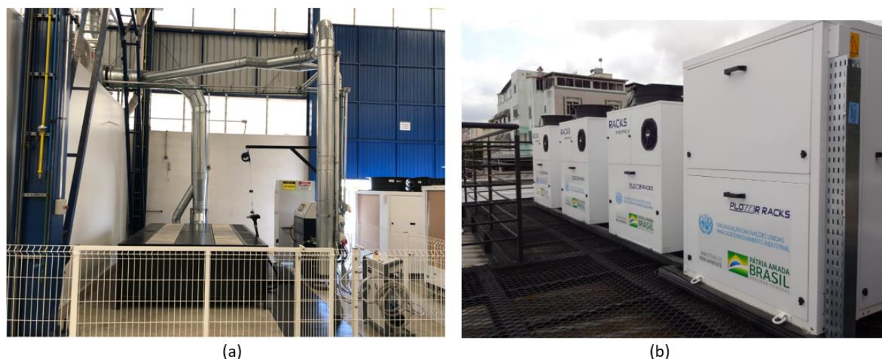
Figure 5 – Filling Line of the Enterprise Plotter Racks (a) and chillers installed by the enterprise at supermarket Bahamas, in Juiz de Fora city (b).
